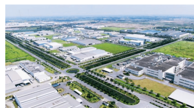
Thang Long Industrial Park II
